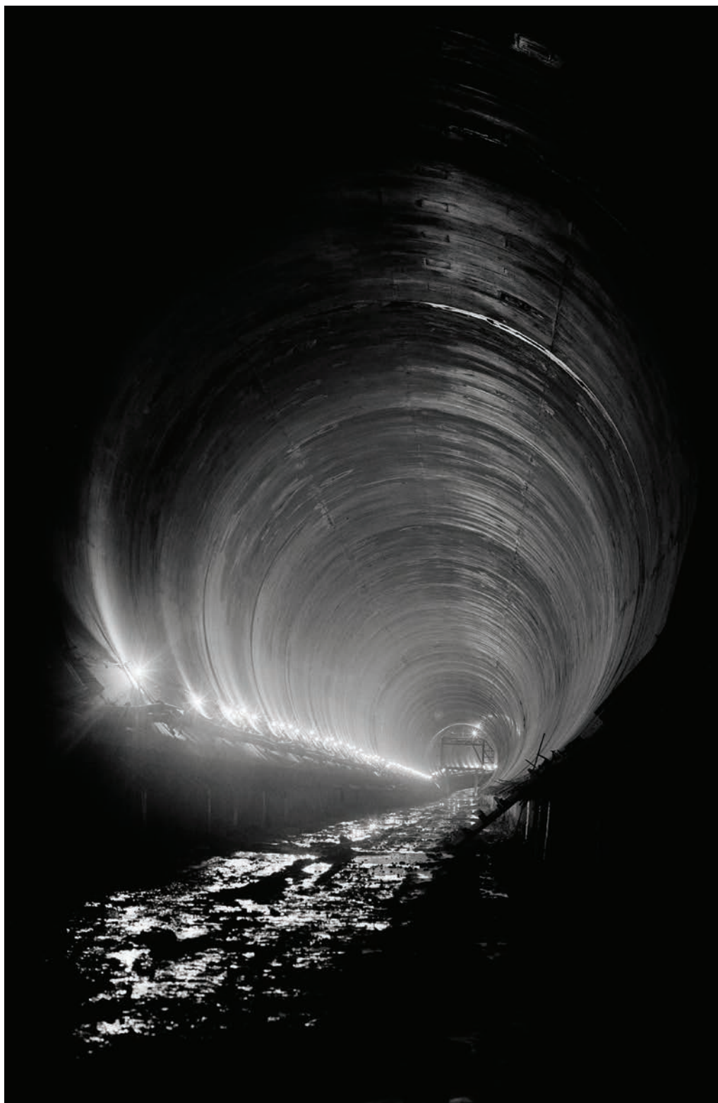
The construction phase of the 35-foot diameter Oroville Dam Diversion Tunnel No. 1 in Butte County, California. Two tunnels were built to divert water from the Feather River during the dam's construction and then plugged at its completion in 1967. Today, the tunnels are used to discharge water from the underground Edward Hyatt Powerplant located near Oroville Dam. Photo taken Aug. 30, 1963. Gene Russell / California Department of Water Resources
