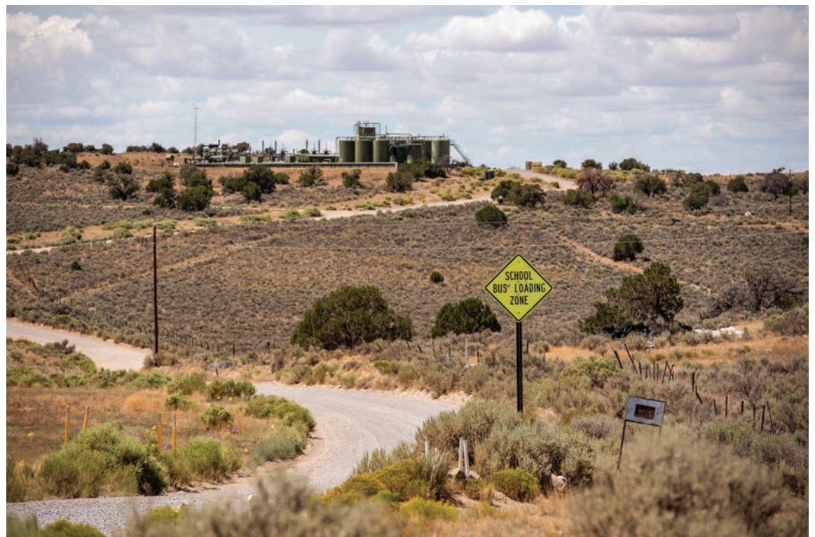
Gas infrastructure near Counselor Chapter's Lybrook Elementary School.
