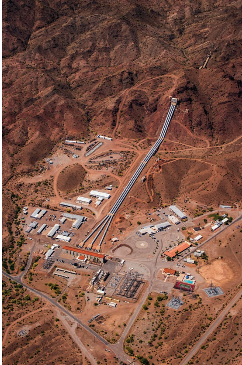
The Gene Pumping Plant near Lake Havasu lifts water hundreds of feet to the Colorado River Aqueduct system, which delivers it to Los Angeles, San Diego and other cities. Southern California gets about 25% of its water from the Colorado River via the aqueduct.
