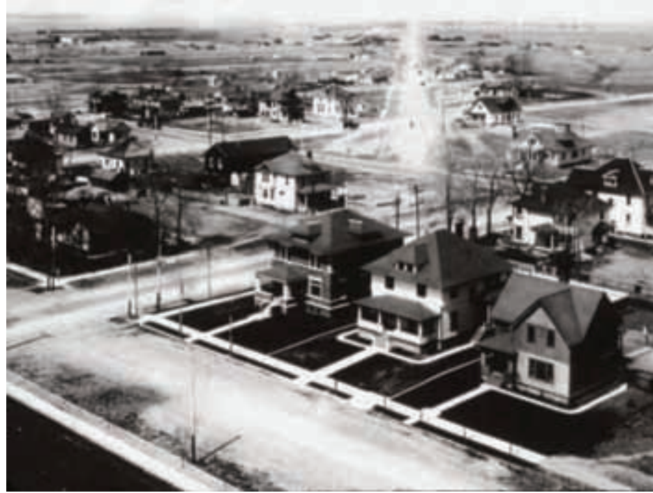
The High Plains transform into a domestic forest of trees and the Herschler Building is built in these photos looking up Randall Avenue in Cheyenne, Wyoming, in 1910 and 2007.
