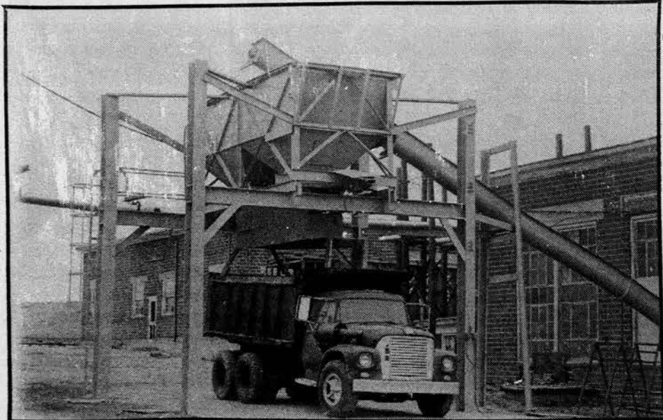
Loading up sewage ash
