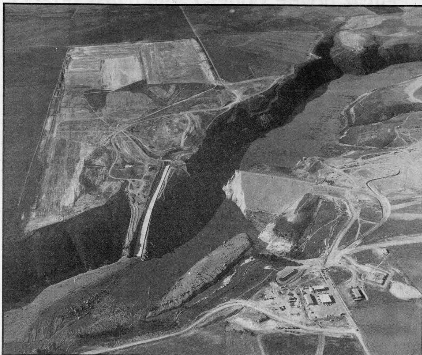
Teton Dam shortly after it failed
