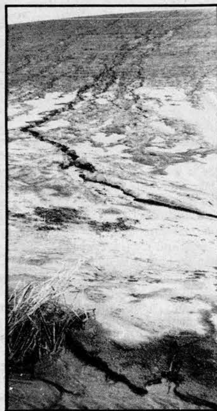
Eroded hillside, Wyoming
