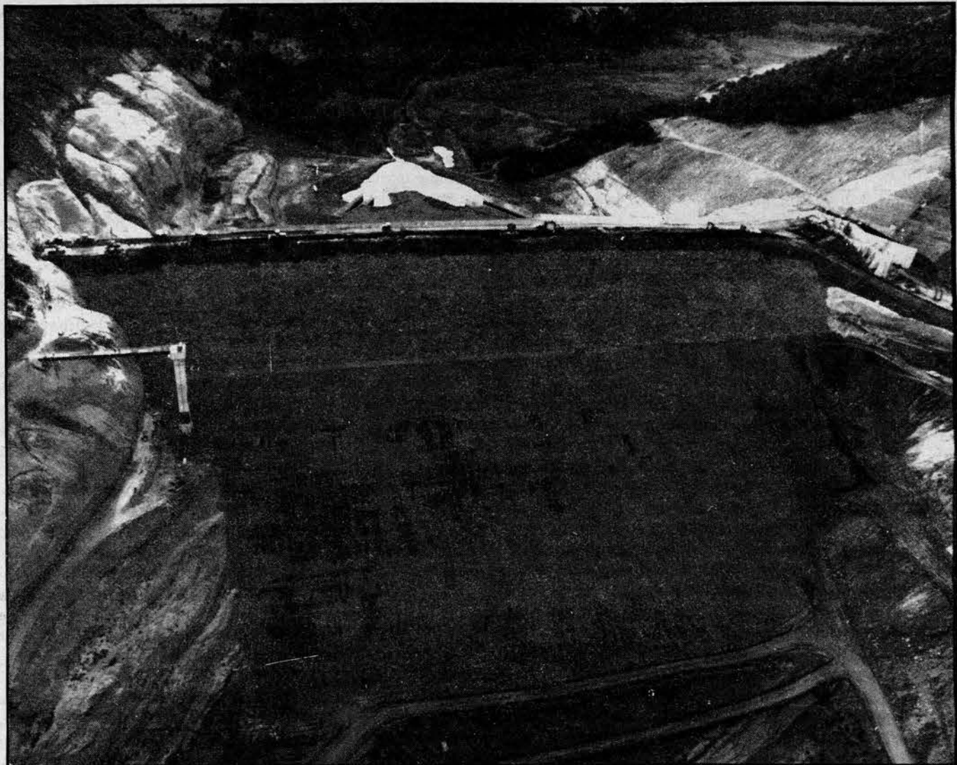
McPhee Dam, nearing completion last summer
