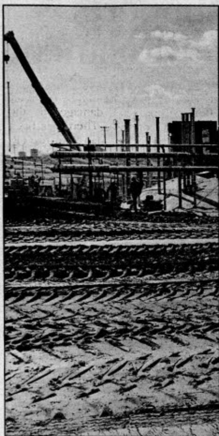
Hanford under construction
