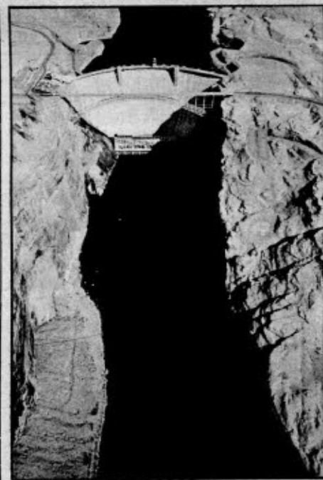
Glen Canyon Dam
