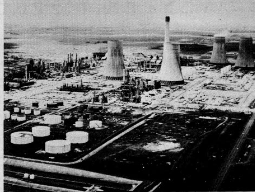
LURGI PROCESS coal gasification is the only commercial-level synthetic fuel process — now in use at two South African plants (one is pictured above). The United States drive toward synthetic fuels is moving from the talking stage to the building stage, or, at least, the spending stage. The $20 billion synthetic fuels corporation legislation will be on the President's desk by next month, according to sources in Congress, where a conference agreement now awaits final approval. And the Department of Energy, which is offering private industry $200 million in grants for feasibility studies on synthetic and alternative fuel plants, reports that it has received 1,000 applications.
