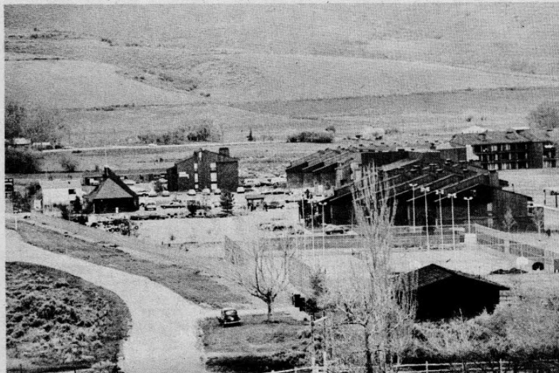
THE RURAL LIFE at Bear Lake fades softly in the path of modern developments. "Own a piece of the water," advertise the owners of this Sweetwater, Inc. complex.
