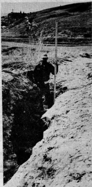
U.S. Soil Conservation Service photo EROSION IN UN-LINED DITCH. The spring run-off in 1960 tore precious topsoil from the sides of this ditch. A metal pipe was later installed, which carries runoff water over the ditch.
