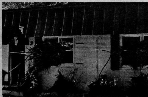
IN A DANGEROUS POSITION. This motel, devastated by the flood in Big Thompson Canyon last July, won't be rebuilt. The Larimer County Commissioners are prohibiting reconstruction of buildings that were more than 50% destroyed by the flood. Photo by Mark Reid
