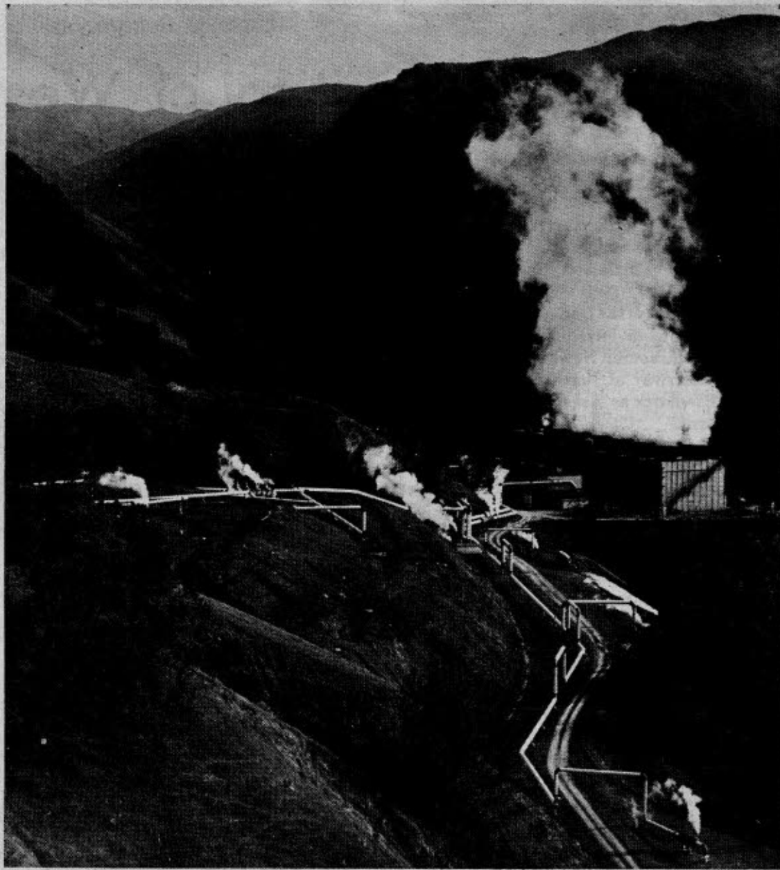
EXPANDING PIPES. Two units of The Geysers power project are shown here with the pipes that feed them steam. Expansion loops allow the pipe to contract when the plant has to be shut down and to expand when the plant starts up. These units, 3 and 4, began in 1967 and 1968 and produce 27.5 megawatts each.
