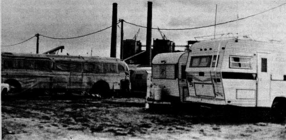
Rock Springs, Wyo. — Pacific Power and Light Co. and Idaho Power Co. are constructing the 2,000 megawatt Jim Bridger Power Plant here. The utilities told Rock Springs officials that the construction force would peak at 1,200-1,250 workers, but in the summer of 1973 nearly 3,000 workers arrived unannounced to the city. Major social problems resulted. Pictured above is a construction camp at the Bridger site. Workers and their families live in buses wrapped in plastic and trailer houses surrounded by mud. No running water, no grass, no yards, no social center. A utility siting act could require that better information be provided to the impacted communities so that they have a chance to prepare.
