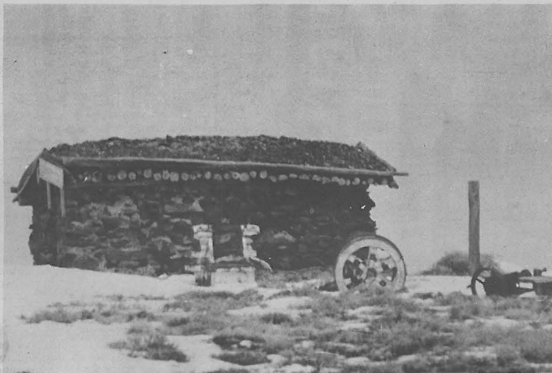
The stone powderhouse sits empty and useless. Here, the dynamite and blasting powder was once stored for use in the hardrock chambers deep underground in the gold mine. This one is located near Atlantic City, Wyoming.
