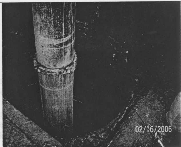
View of cellar with conductor pipe and mouse hole pipe while facing southeast at ground level in the substructure rig 455
